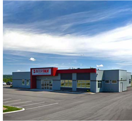
371 CUTLER AVENUE SINGLE TENANT BUILDING DARTMOUTH
