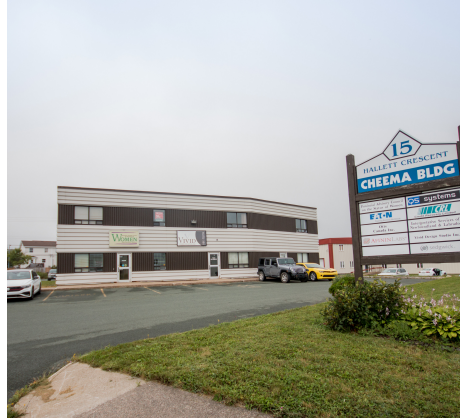
15 HALLETT CRESCENT CHEEMA BUILDING ST. JOHN'S
