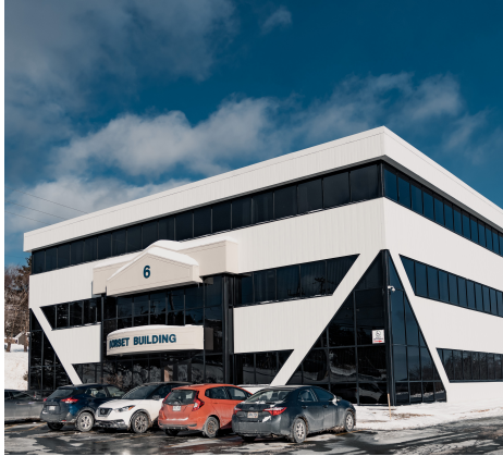
6 MOUNT CARSON AVENUE DORSET BUILDING MOUNT PEARL
